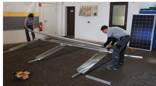
FIGURE 5: FLAT ROOF PV MOUNTING SYSTEM EXAMPLE.
