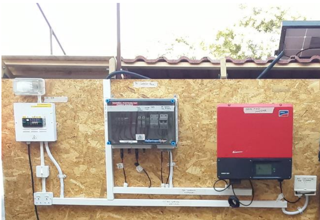
FIGURE 3: EXAMPLE TRAINING INVERTER INSTALLATION
