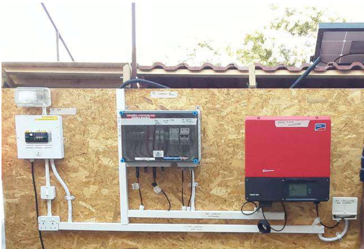
FIGURE 10: COMPLETED INSTALLATION TO BE ASSESSED
